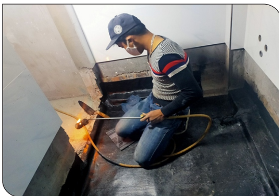
Construction of torched on membrane
